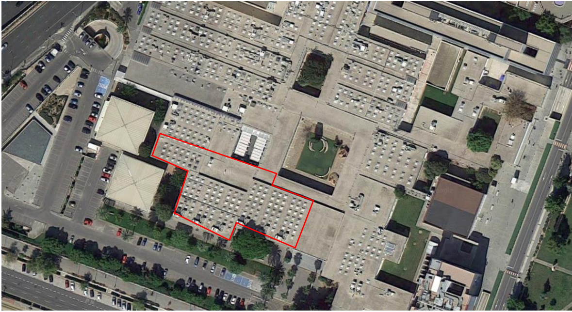
Fig. 1.2: Picture of the location of 'area 4' at ETSIE Building
