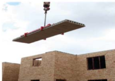
Fig. 3 Installing hollow core strip slabs.
