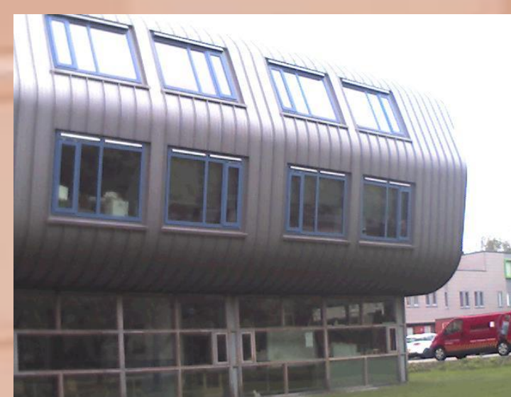
Heat bridges at the windows and in some points at the facades
