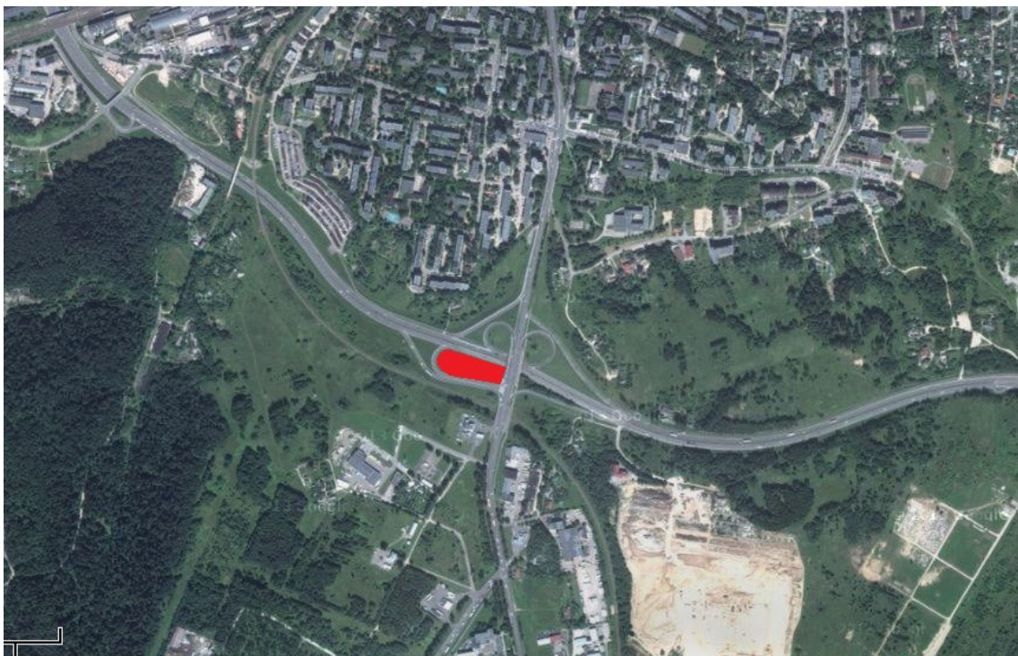
Figure 1.3. Aerial view of construction site
