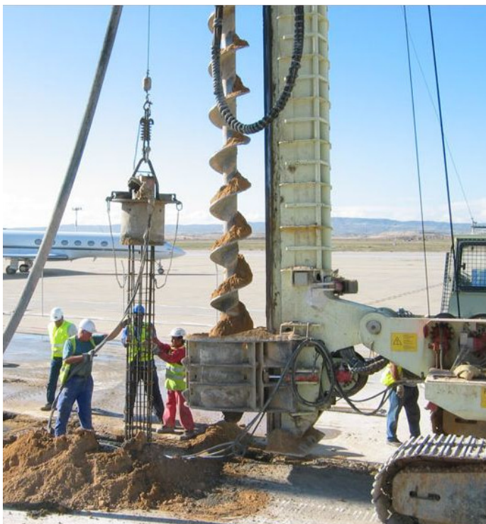
Figure 2.2. Pile drilling
