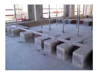
Boyd beam reinforced with metal bars and concrete
