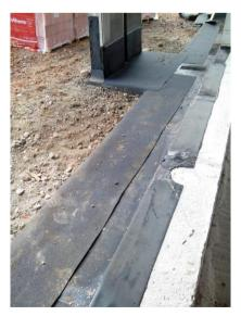
PIR insulation and polyethylene membrane (retaining walls)
