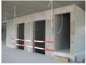
Precast/bearing walls in the lift and stairs module
