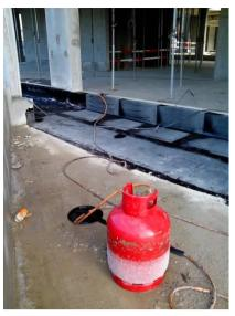
Bitumen membrane applied with torch
