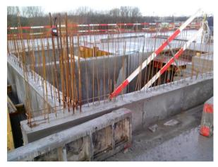
Metal bars to connect cavity walls
