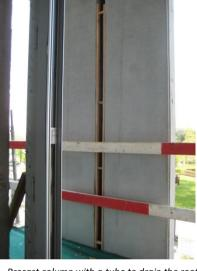
Precast column with a tube to drain the roof
