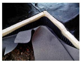
PIR insulation and polyethylene membrane (retaining walls)
