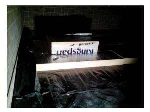
PUR insulation and PE sheet in the basement
