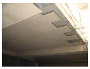
Acoustic and thermal insulation panels "stertekt" for ceilings in the basement
