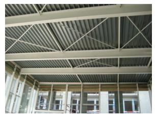
Universal beams and rectangular hollow profiles that hold the roof
