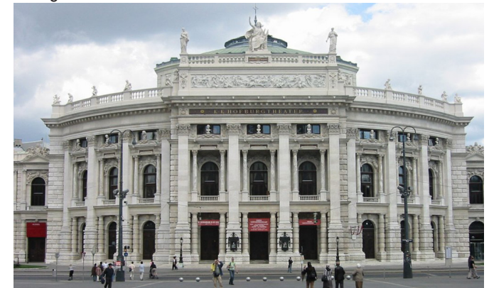
Fig. 54. Vista general del Burgtheater.
