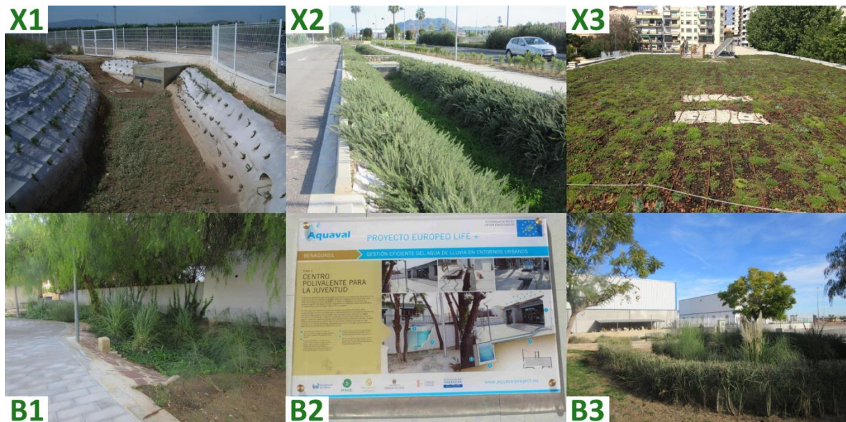
Fig. 1. Showcase sites after SuDS development/retrofitting in Xàtiva (upper row) and Benaguasil (lower row).
