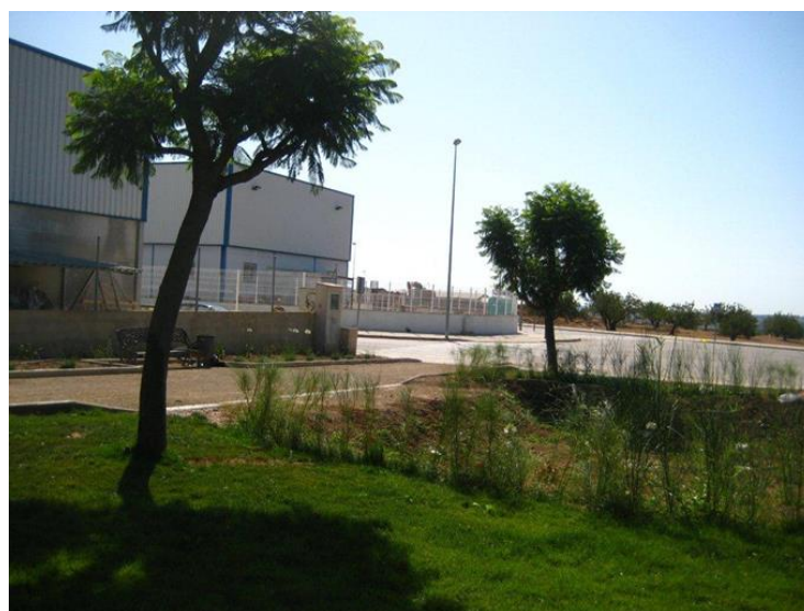
Run-off disconnected to a nearby retrofitted detention-infiltration basin in Benaguasil (Valencia).
