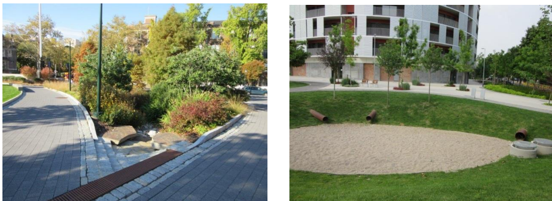
Figure 1. Rain garden in Philadelphia (left); infiltration basin in Barcelona (right).
