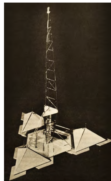
Tokyo (Shoriki) Tower, R.B. Fuller, 1966
