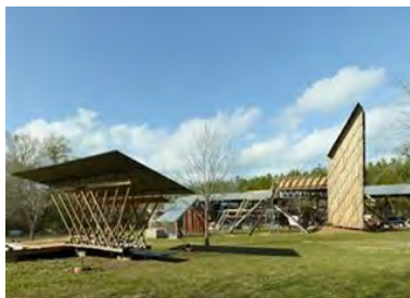
Tinnings Bathhouse, Rural Studio, 2011
