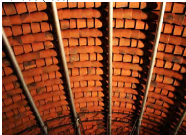
Wall House, Auroville, India, Anupama Kundoo (2000)
