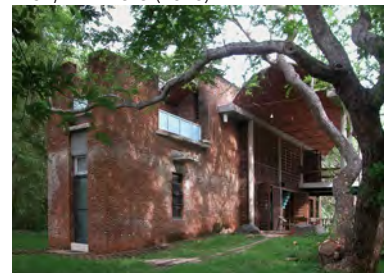
Wall House, Auroville, India, Anupama Kundoo (2000)
