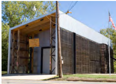
Newbern Fire Station, Rural Studio, 2004
