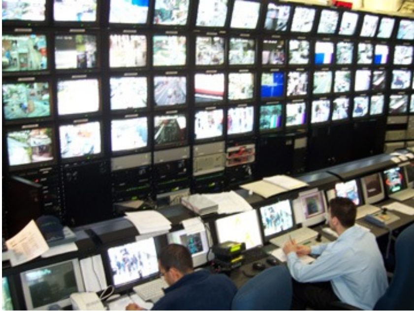
Figure 1.1: An example of CCTV control room at United College [operators].
