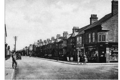
3.204_Wolverton, Stradford road, 1930
