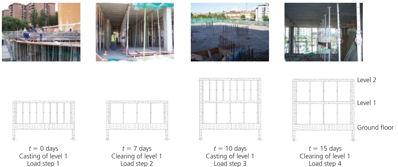
Figure 2. The construction process from start to day 15
