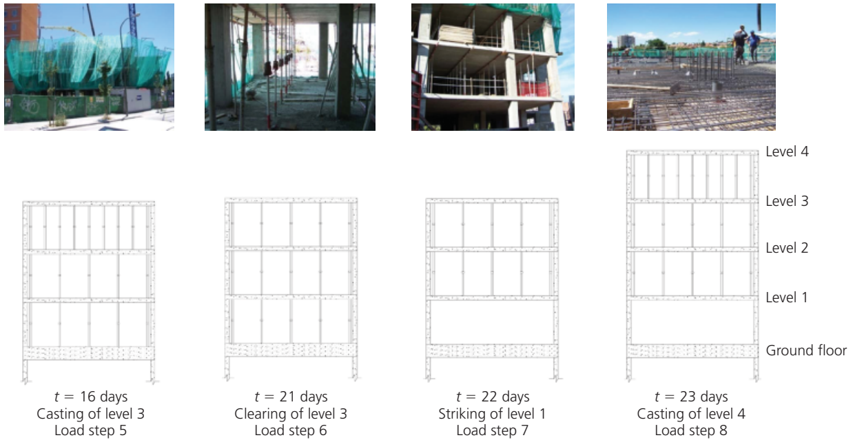
Figure 3. The construction process, day 16 to day 23
