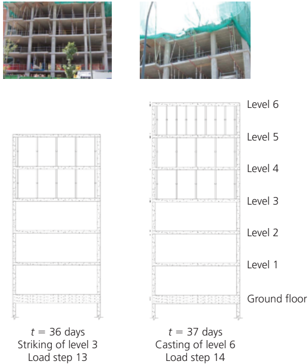
Figure 5. The construction process, days 36 and 37
