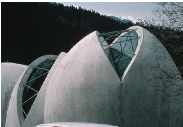
Figure 5: Evangelical Church, Cazis, Switzerland (1996). Photograph: Heinz Isler
