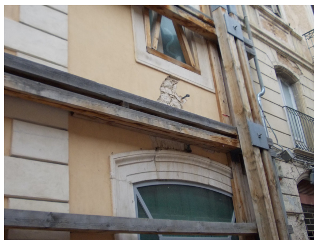
Fig. 17 _ Variation of discoloration in function of exposure to sun and rain and constructive positioning
