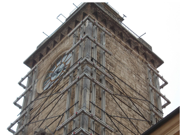
Fig. 14 _Total hoop with mixed system
