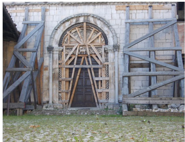
Fig. 4 _Wooden retention shoring
