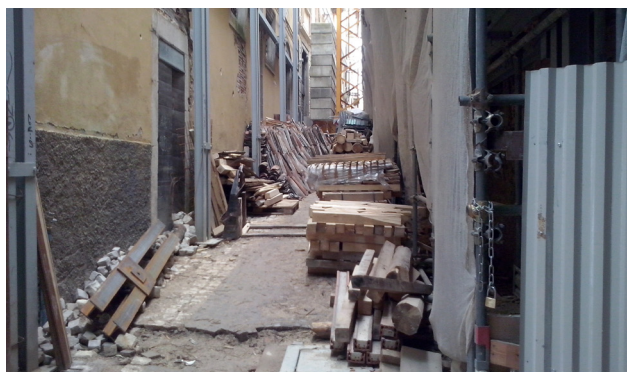
Fig. 3 _Occupation of the road with reconstruction site
