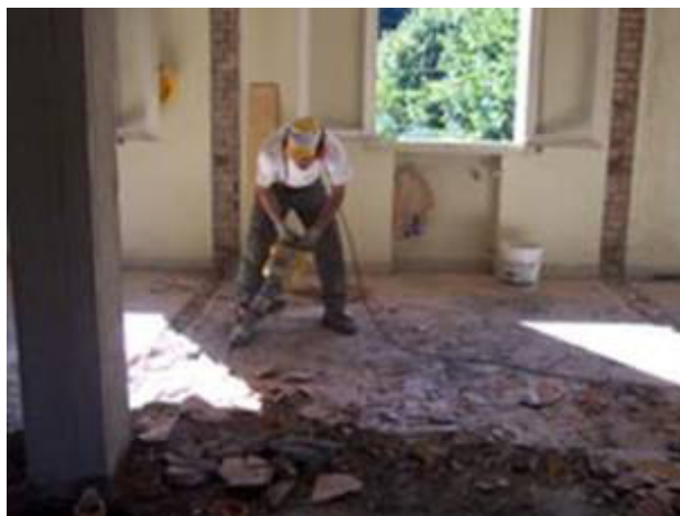
Fig. 11 _ Centro Porretta Terme. Demolition of flooring and subfloor with a jackhammer.
