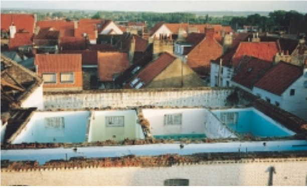
Fig. 6 _ Residence Taviel, deconstruction for each floor
