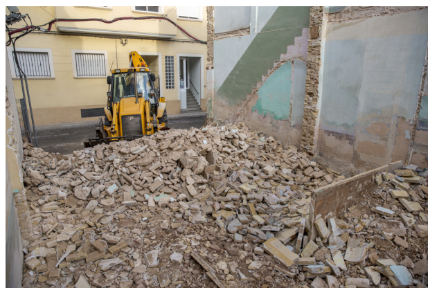
Fig. 23 _Debris removal with mechanical means
