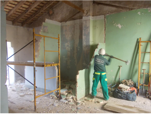
Fig. 19 _Demolition of internal partitions with a hammer
