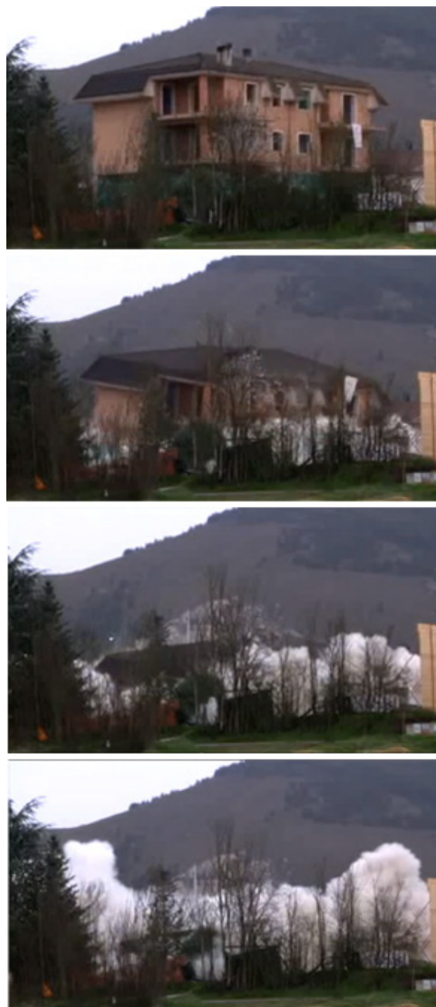
Fig. 4 _ Demolition with explosive charges (AQ)
