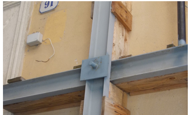
Fig. 38 _Uprights and crossbeams single welded UPN profiles
