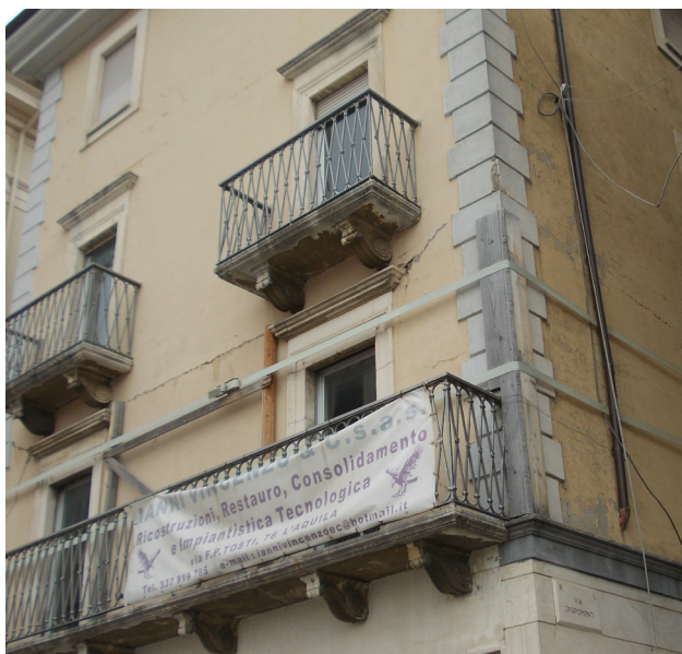
Fig. 43 _Hooping of a building with polyester bands
