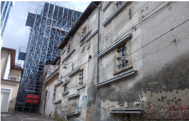
Fig. 33 _Crossbeams UPN coupled profiles
