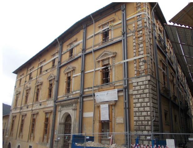
Fig. 17 _Inner passing tie rods
