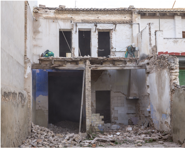
Fig. 20 _Demolition of the additions.
