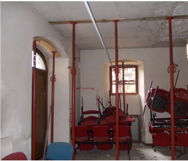
Fig. 10 _Support shoring with props
