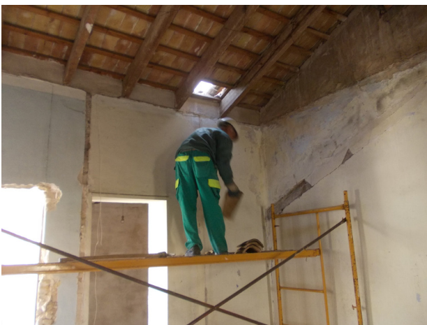
Fig. 21 _Initial phase of dismantling the roof.
