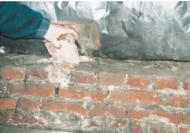
Fig. 7 _ Residence Taviel, manual deconstruction of the wall
