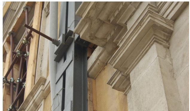
Fig. 37 _Uprights HEA coupled profiles
