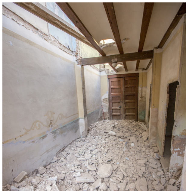
Fig. 22 _Demolition of intermediate floor
