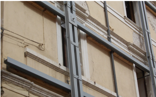
Fig. 34 _Crossbeams single HE profiles, uprights HEA coupled profiles
