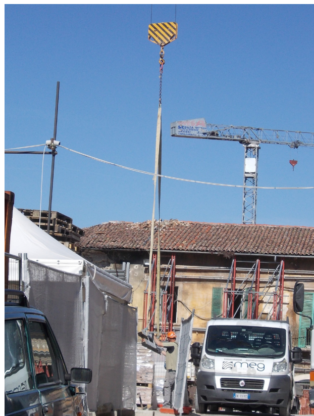
Fig. 22 _ Dismantling the steel grid
