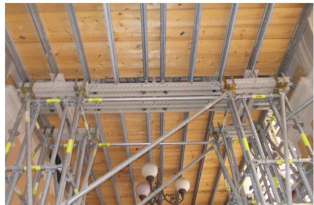
Fig. 24 _Details of support shoring, L'Aquila, Corso Vittorio Emanuele, april 2013
