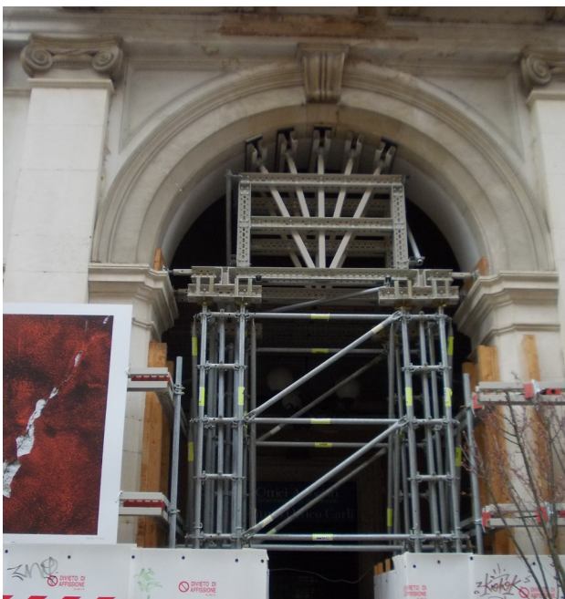
Fig. 11 _Centering with multidirectional system
