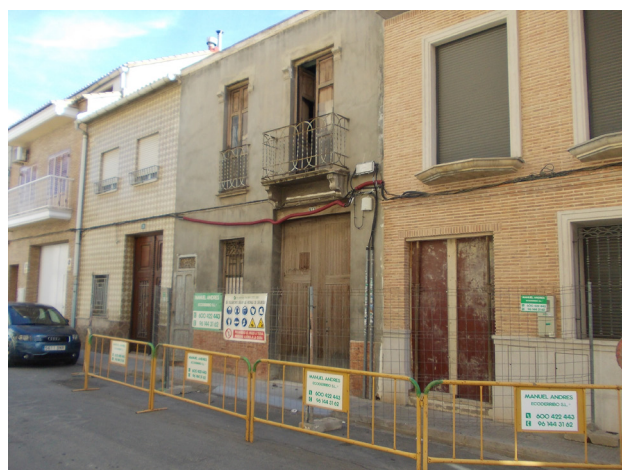
Fig. 17 _Front view of building located in Massamagrell
