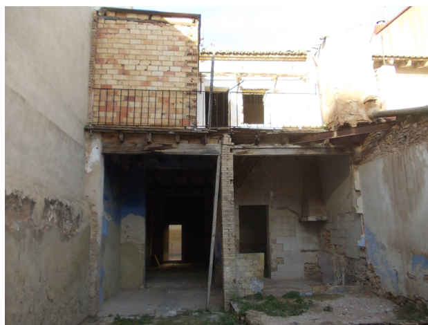
Fig. 18 _Rear view of building located in Massamagrell
