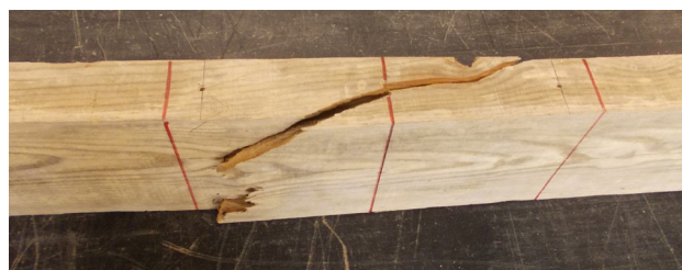
Fig. 15 _Structural failure of element n.8, view frontal
