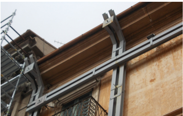
Fig. 35 _Uprights and crossbeams HEA coupled profiles
