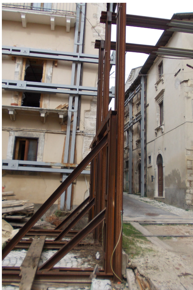
Fig. 26 _Metallic carpentry with welded profiles
