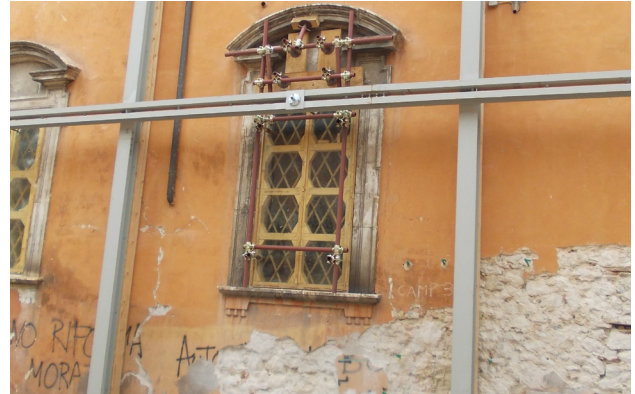
Fig. 36 _Uprights HE, crossbeams couples UPN profiles
