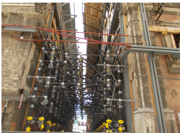
Fig. 7 _Counteracting shoring with tubes-clamps system
