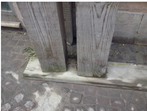
Fig. 21 _ Attack animal of uprights in the point of contact to the ground
