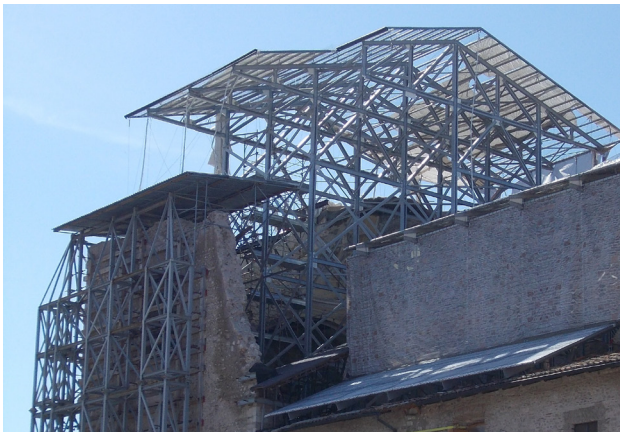
Fig. 19 _Cover with steel structural profiles
