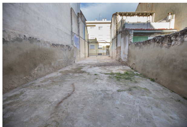
Fig. 24 _Area after the demolition
