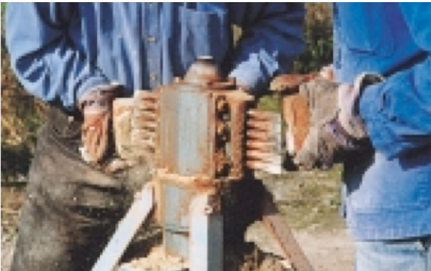
Fig. 8 _ Residence Taviel, manual cleaning of the bricks
