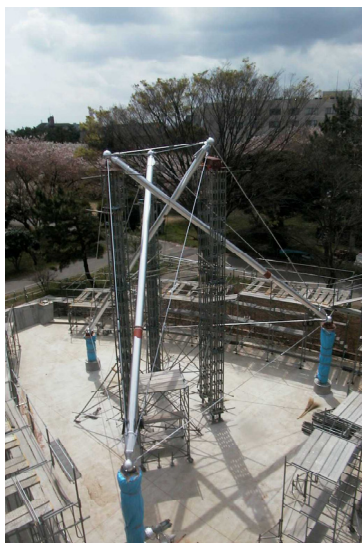
Figure 2. Frame A under construction
