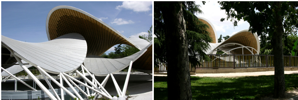
Figure 11 Auditorium after completion of the structure
