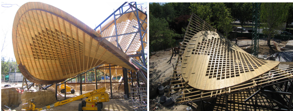
Figure 9: Temporary Support Structure and first layer placement
