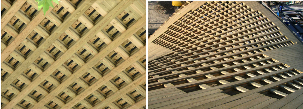
Figure 4: Timber planks arrangement views from under and over the structure
