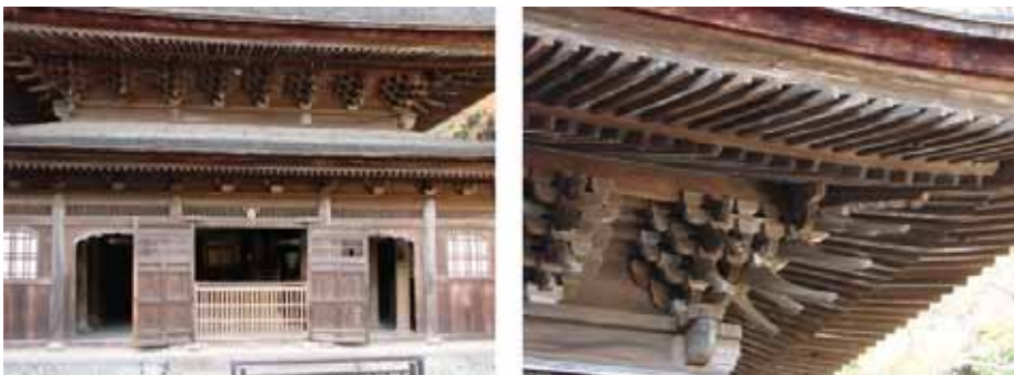
Figure 8: 3 stepped bracket complex to support overhanging eaves
