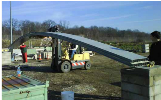
Figure 12. Positioning of the beam on its final position
