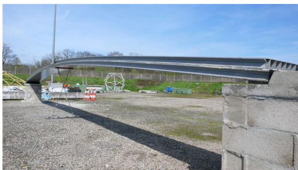
Figure 15. View of the complete footbridge
