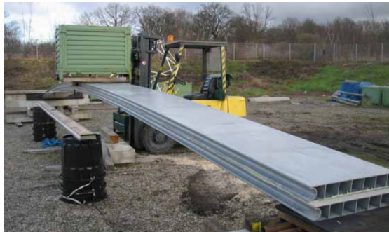
Figure 13. Loading of the beam in order to set up the cable
