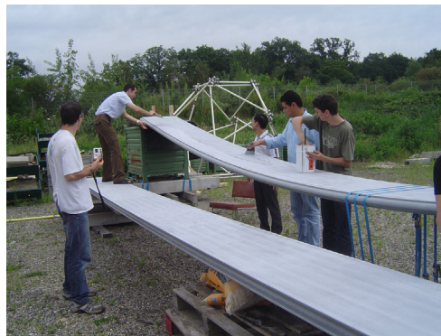
Figure 10. Preparation of the bonding
