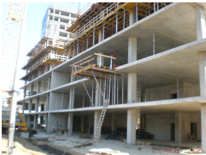
Figure 2: The building under construction
