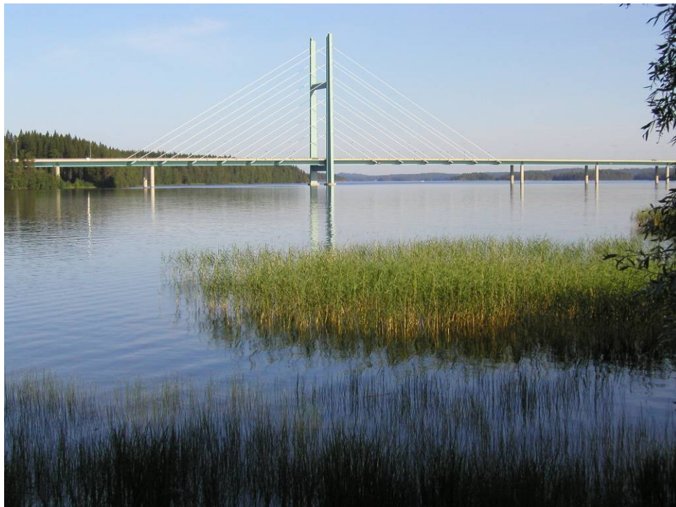
Figure 2. Tähtiniemi Bridge in summer.
