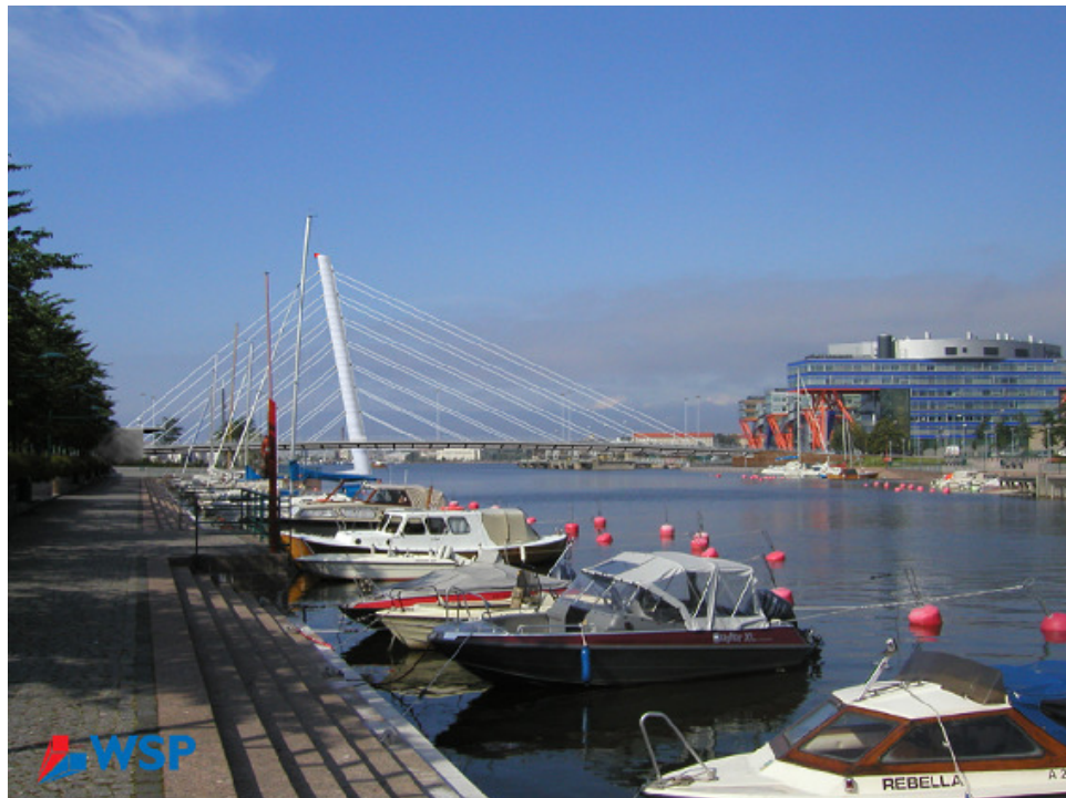
Figure 5. Crusell Bridge in photo montage. The bridge is now under construction.
