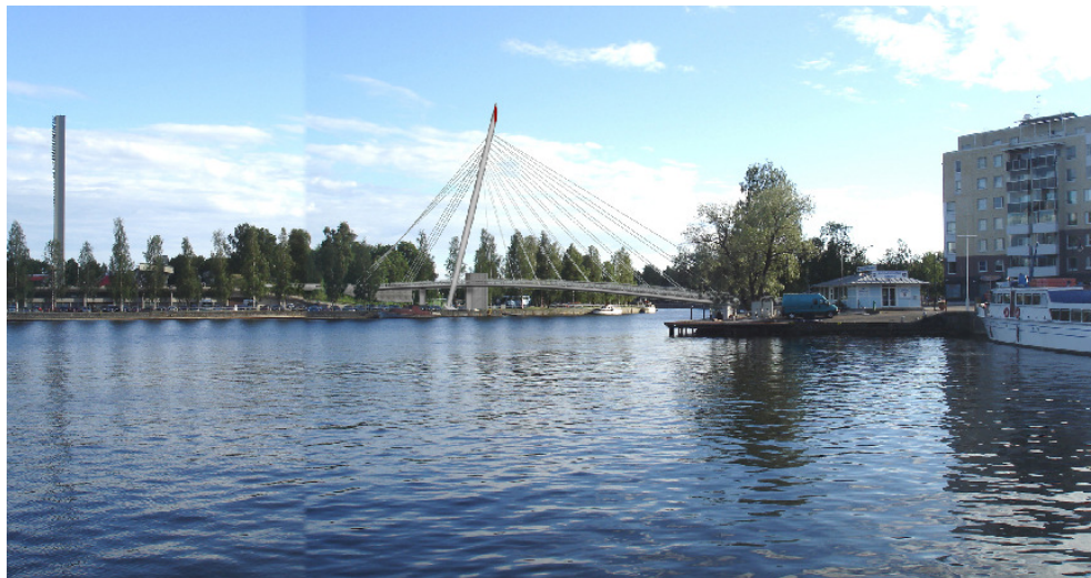
Figure 7. The winner of Laukko pedestrian bridge design competition. The bridge is under construction.
