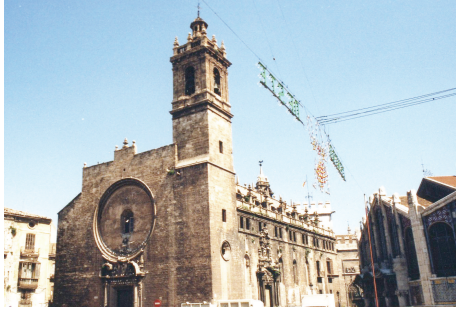
FIGURE 1: Overview of the church of Santos Juanes .
