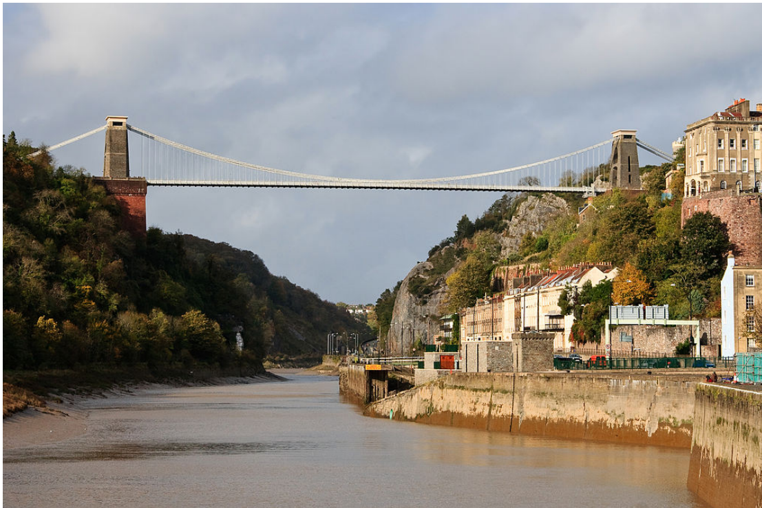
Figure 7. The southern side of the Clifton Suspension Bridge with Avon Gorge in the background. The Leigh Woods tower (left) has a different design to that of the Clifton tower (Gothick, 2009).
