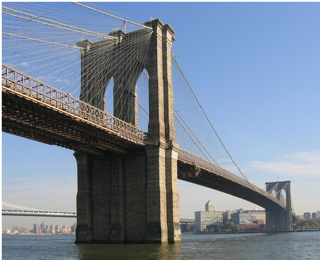
Figure 1. The Brooklyn Bridge, with vertical hangers and inclined stays visible (User:Postdlf, 2005).
