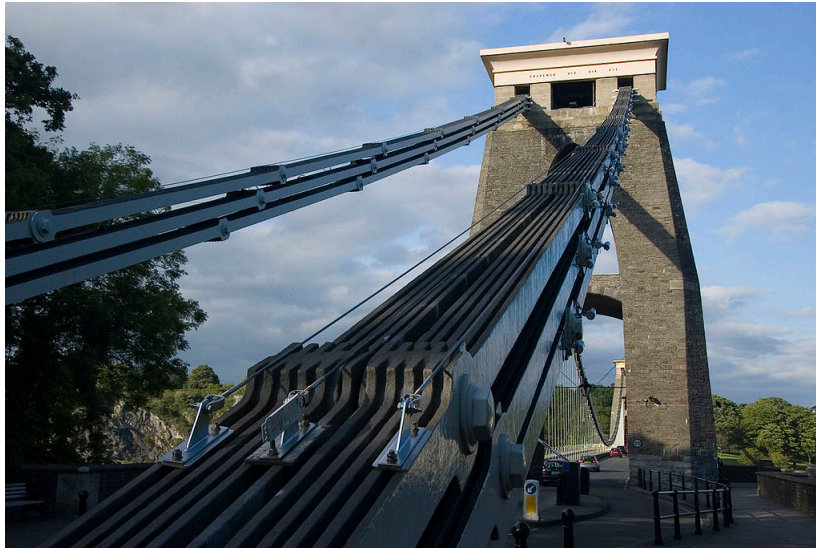
Figure 10. Photograph of the Leigh Woods tower with the land chains in the foreground (D, 2007).
