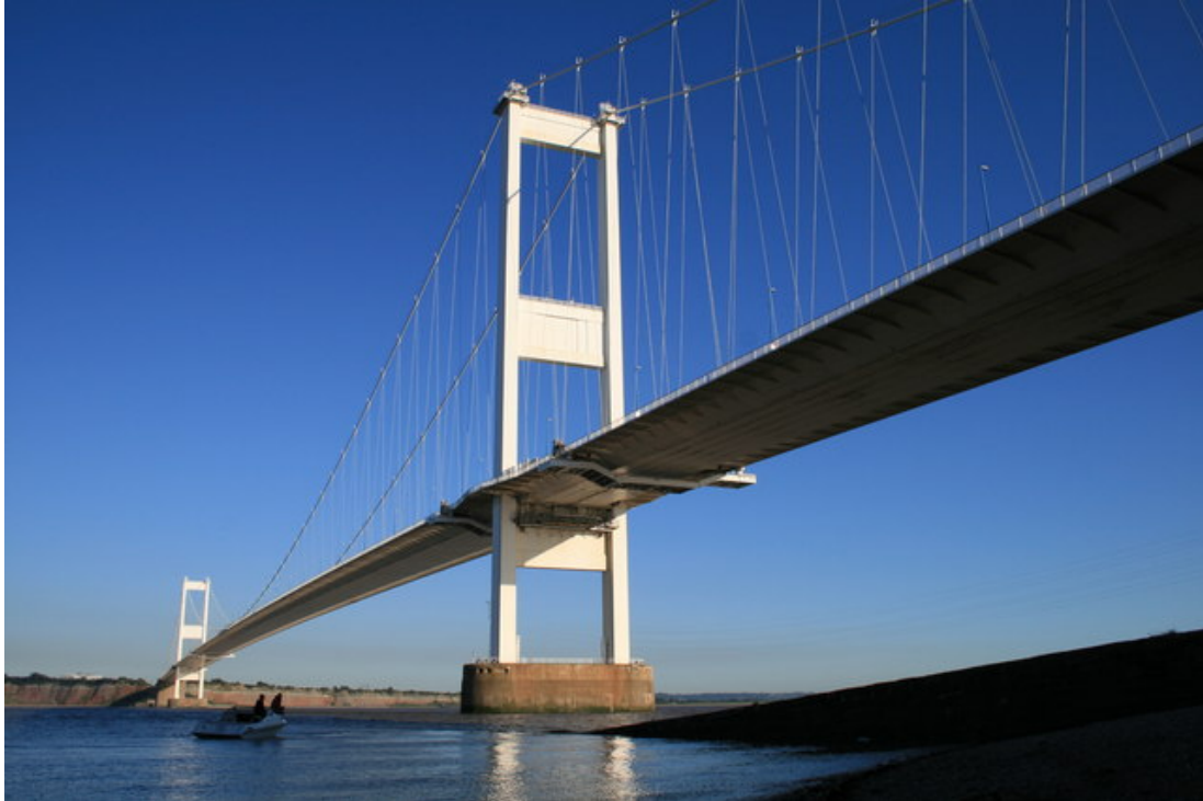
Figure 3. Photograph of the Severn Bridge, showing inclined hangers and aerodynamic deck profile (Edwards, 2007).
