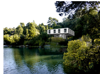
GUNA HOUSE San Pedro, Chile 2010-2012, Under construction
