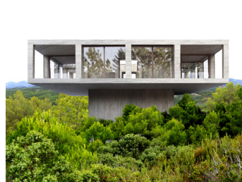
SOLO HOUSE Cretas, Spain 2009-2012, Under construction
