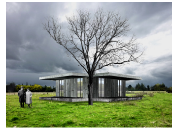
ABBA HOUSE Cabrero, Chile 2011, Under construction
