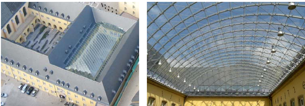
Figure 7: Glazed Roof over the main courtyard of the Neumunster Abbey
