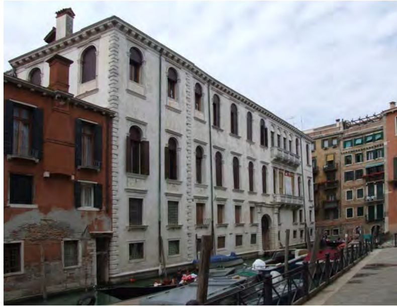
Fachada al canal de San Severo en 2008, tras la restauración (foto Claudio Menichelli) Facade on the Rio di San Severo in 2008, at the end of the restoration (photo Claudio Menichelli)
