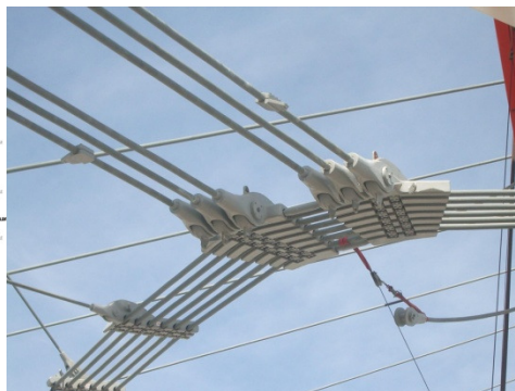
Figure 11a. Simplified detail drawing Figure 11b. Casting at tension ring of 3 tons each
