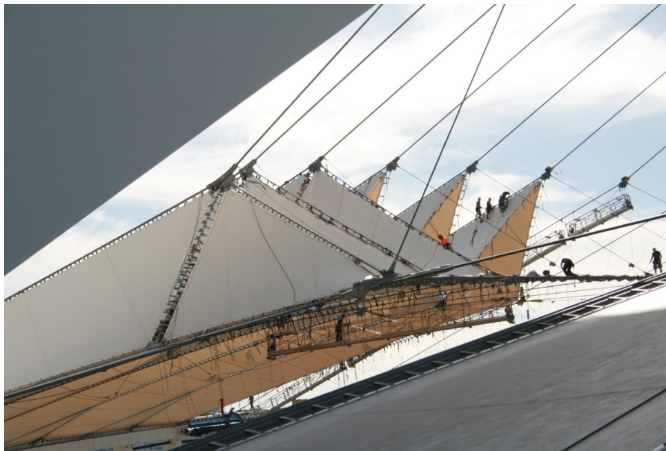
Figure 15: Installation of membrane panels between ridge and valley cables
