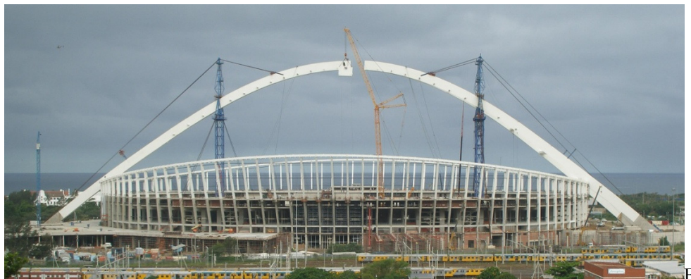
Figure 14: Arch structure supported by towers and backstays
