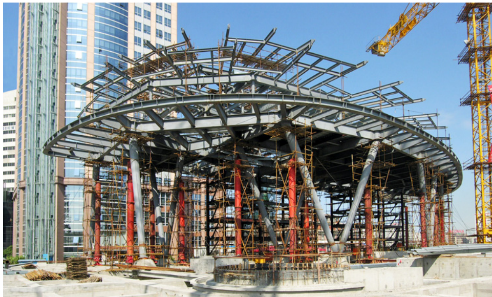
Figure 7: Steel platform and floors erection
