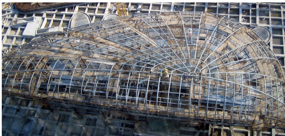
Figure 8: Steel framed roof installation
