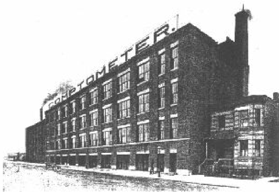
Modern Reinforced Concrete Factory Recently Built for Manufacturing Comptometers
