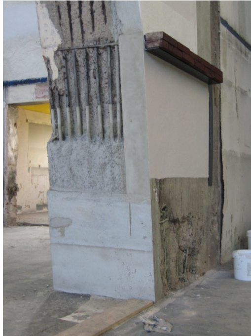
Figure 9: Principles of renovation, tested at one column
