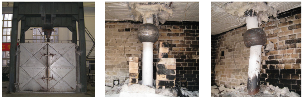
(a) Fire-Resistant test equipment (b) Joint before the test (c) Joint after the test Figure 3: Fire performance test on the welded hollow spherical joint
