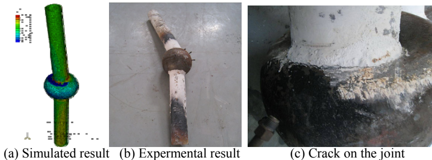
Figure 5: Failure modes of the first joint
