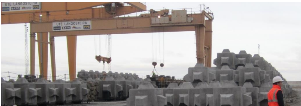
Figure 5.4 Cubipod ® block yard with gantry cranes (Port of Punta Langosteira, Spain).
