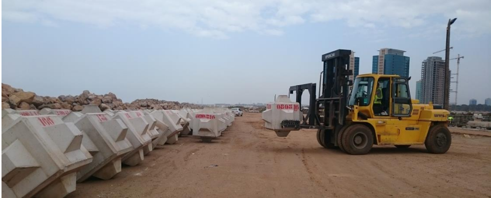
Figure 5.5 Block yard of 3-tonne Cubipod® units handled with a forklift (Marina Bay D'Alger, Algeria).
