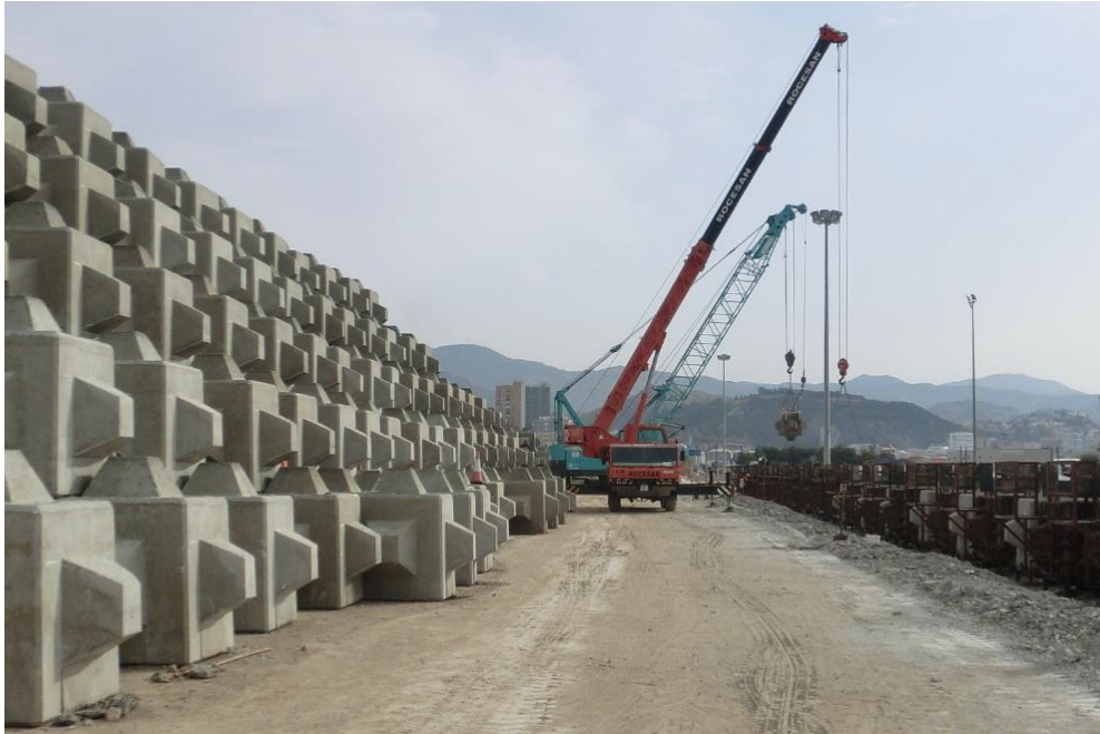
Figure 1.9 Five-level stacking of Cubipod ® units (Port of Málaga, Spain).
