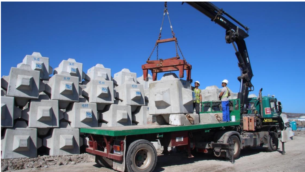
Figure 5.6 Block yard of 6-tonne Cubipod® units handled by a boom truck (Port of Las Palmas, Spain).
