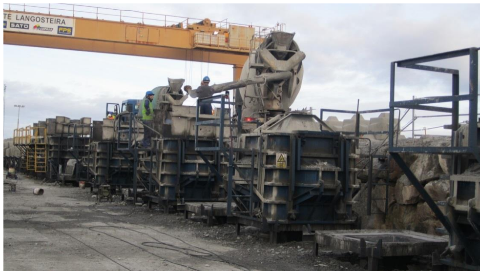
Figure 1.7 Concrete being poured into the molds to manufacture 25-tonne Cubipod ® units.
