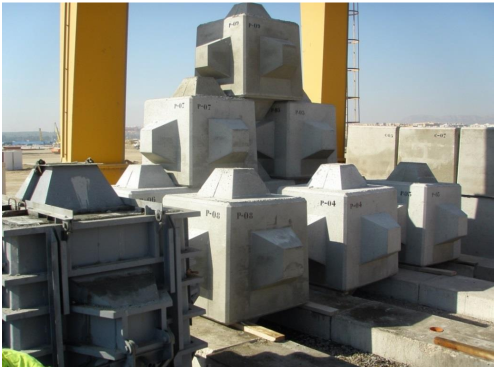
Figure 1.3 Fifteen-tonne cube and sixteen-tonne Cubipod ® units in the Port of Alicante (Spain).
