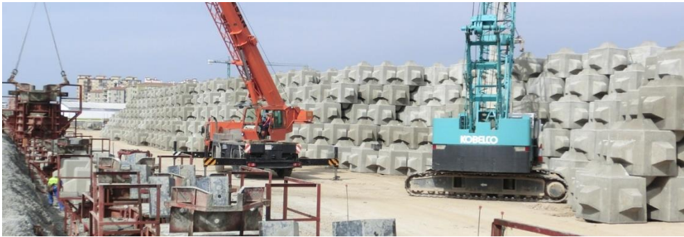
Figure 5.3 Five-level stacked Cubipod ® units in the block yard (Port of Málaga, Spain).
