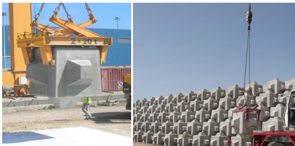
Figure 5.2 Double pressure clamps handling Cubipod® units in the block yard.
