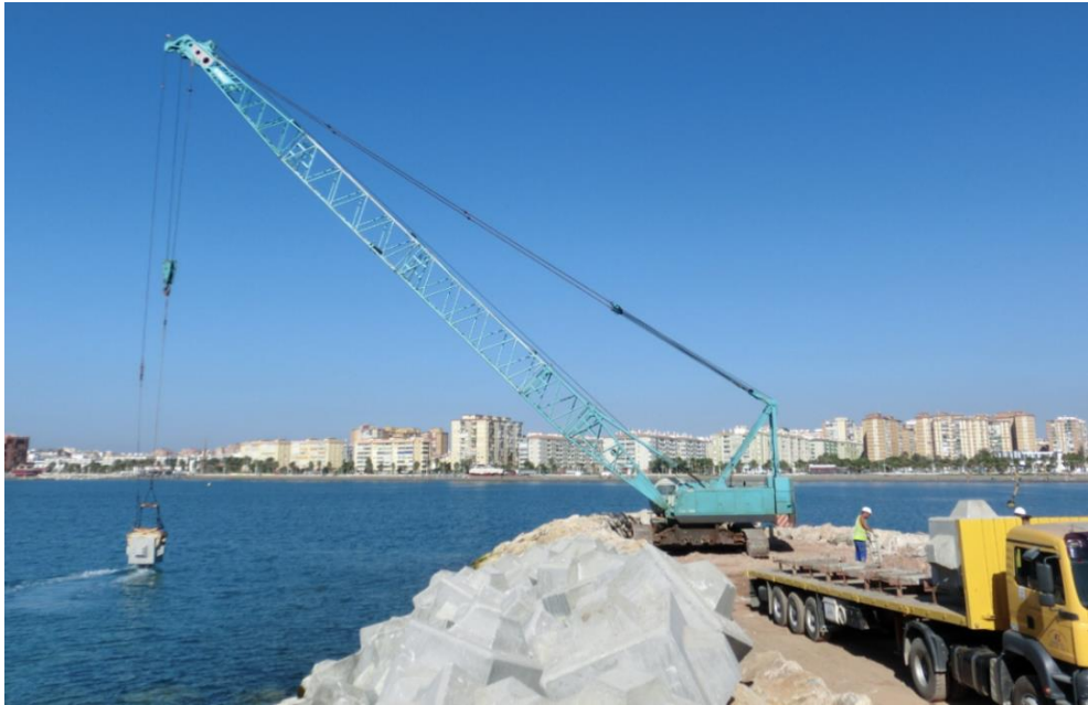
Figure 6.2 Placing Cubipods in San Andrés Breakwater (Port of Málaga, Spain).
