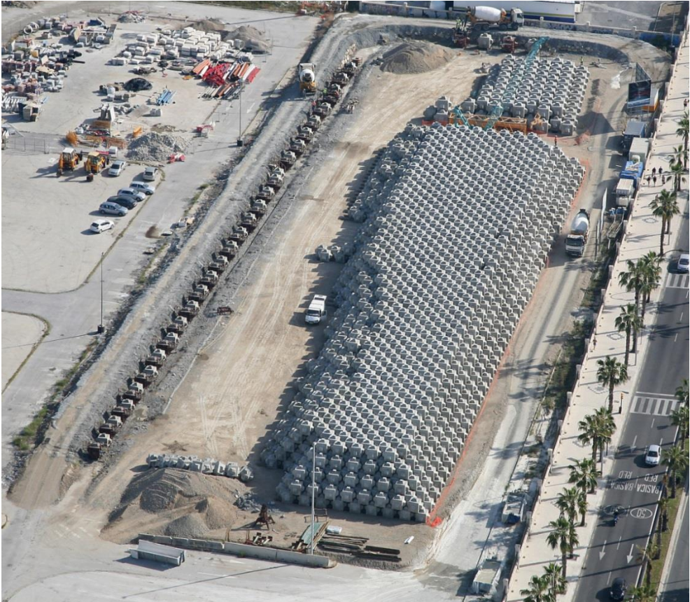
Figure 5.11 Extensive Cubipod ® block yard with wheeled cranes at the Port of Málaga (Spain).
