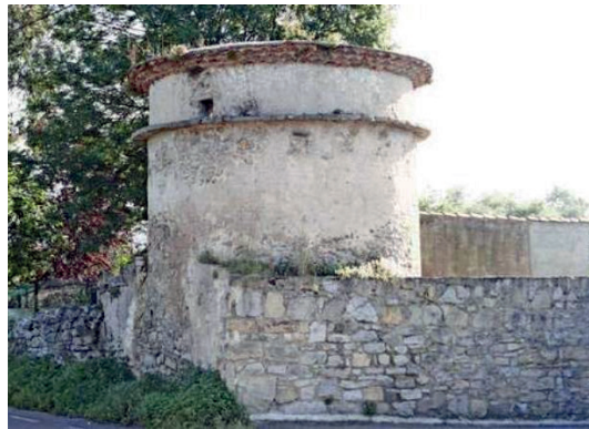
Figure 7. Palomar in Pedrera road (Porceyo).
