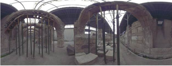
Figure 16: Metal stands to strenght abutments.
