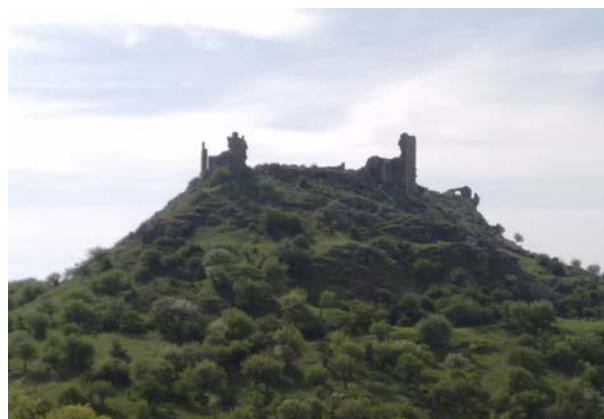
Figure 2: General outer view of the castle of Uggiano (Ferrandina, Basilicata, Italy).
