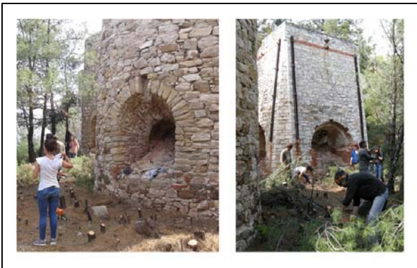
Figure 4: The kilns during vegetation removal.
