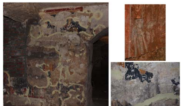
Figure 3: Eastern wall of Room I (Oratory C, Region C): Fresco of the Little Commissioner.
