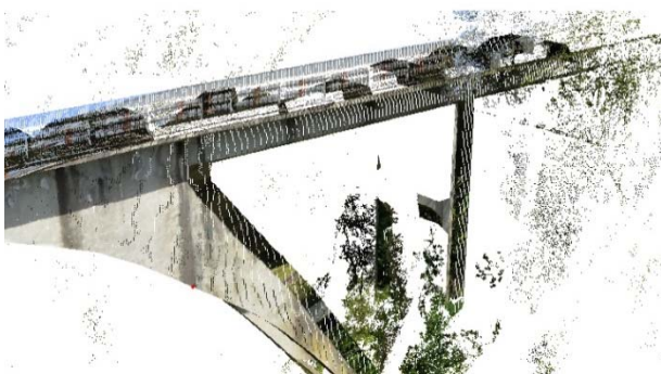
Figure 2: Top: Union of scans. Bottom: detail of a colored point cloud.
