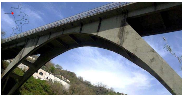
Figure 1: The Caprovidi bridge.
