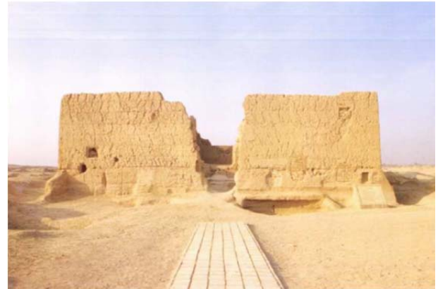
Figure 3: Northwest Small Temple after restoration on site (UNESCO Beijing office 1999).
