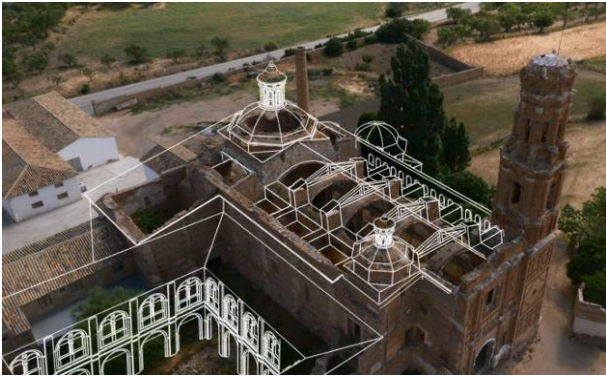
Figure 16: 3D model with wireframe view overlaid over the real image of the building.
