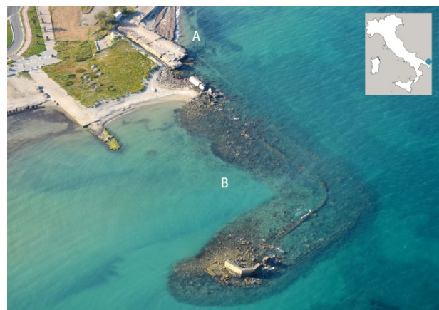
Figure 1: General aerial view of the ancient harbour at St. Cataldo. A: the roman pier; B: the new breakwater.
