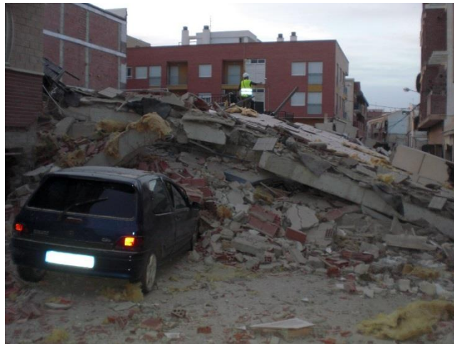
Figure 1: Building failure in Lorca earthquake (Spain, 2011)
