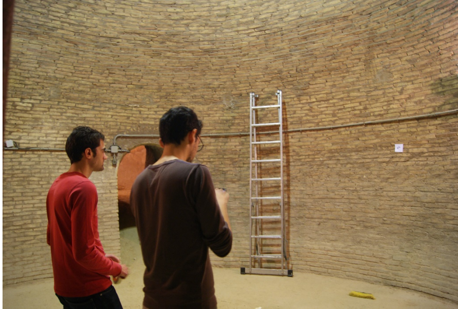
Figure 68. Placing targets in the silo 2.
