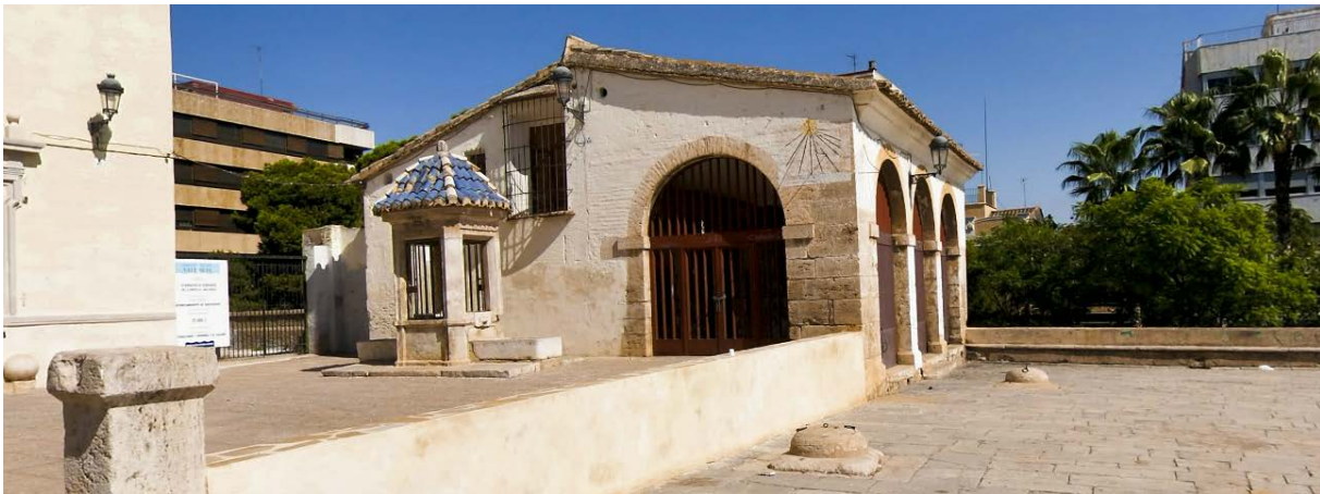
Figure 19. View of one of the building called " embarronat " 7 . 2016.
