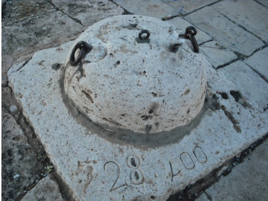
Figure 13. Cap of the Silo number 28, with a capacity of 400 cahíces . 2016.
