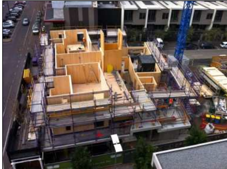
13. Picture of the Forté under construction source: http://www.thefifthstate.com.au/articles/ct-could-spark-local-manufacturing-industry/51883
