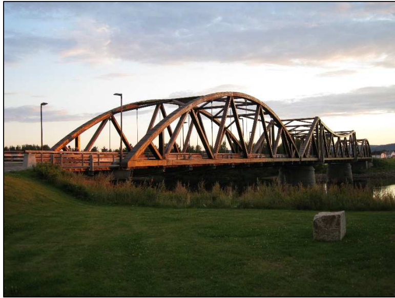
7. Flisa bridge 200 length – source: BROR.NO
