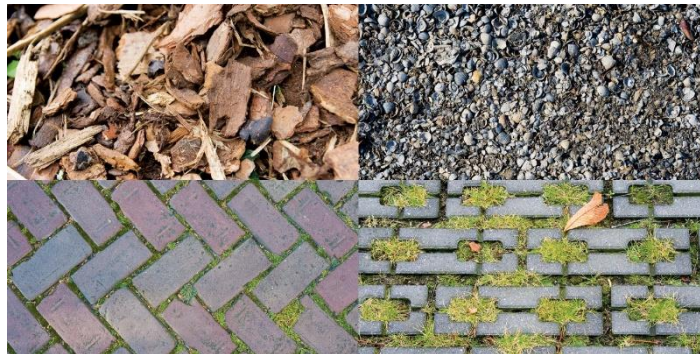
Figure 6 Different types of porous paving materials
