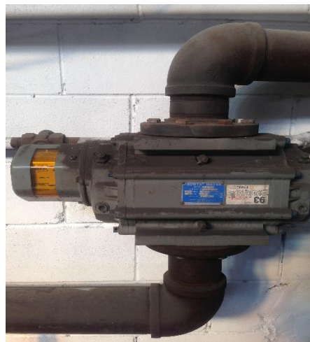
Image 40 DRESSER Series B3: 11M175 ROOTS gas meter
