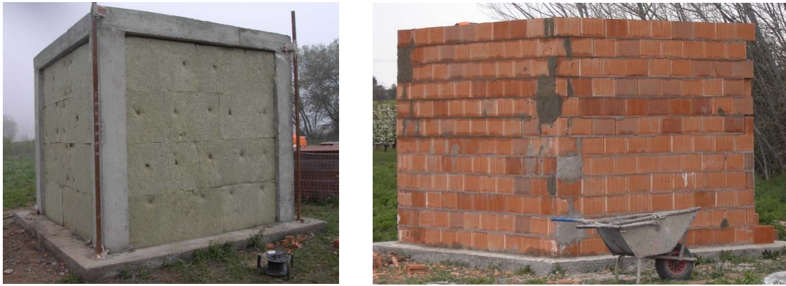
Figure 1. Cubicles of the experimental campaign. Insulated cubicle (MW, left) and inertial cubicle (ALV, right).
