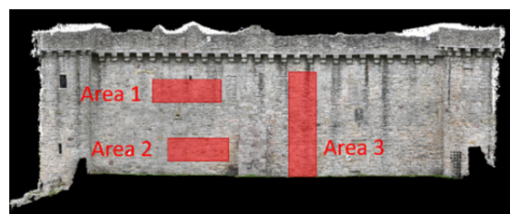
Figure 3: The three areas within the East rampart wall that are used for the assessment of performance in terms of accuracy and precision.
