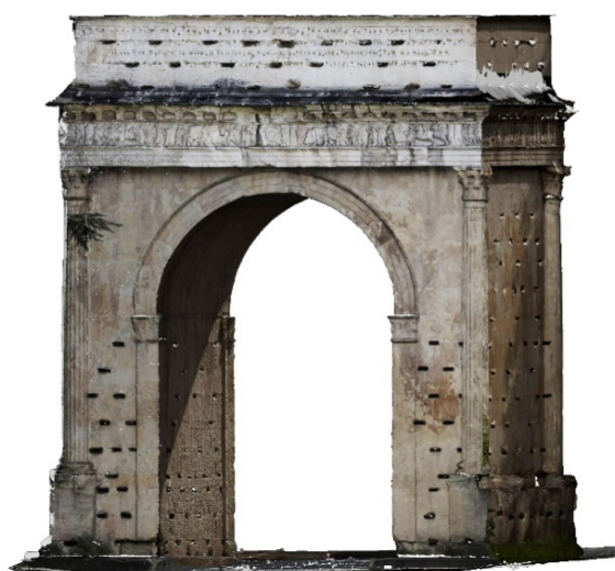
Figure 1: Integrated photogrammetrical and laser scanning model of the Arch of Augustus.
