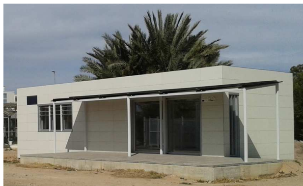
Figure 1. Case study constructed building
