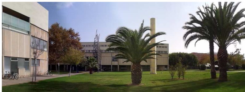
Figure 8. West-east view of the future building location.
