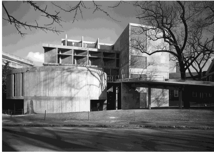
12. Le Corbusier, Visual Arts Center, View from Quincy Street © Fondation Le Corbusier-ADAGP, 2015).
