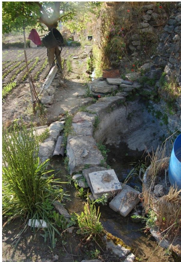
Fig. 8. The semicircular cistern in the vegetable gardens of the Vallone dei Lavandari.
