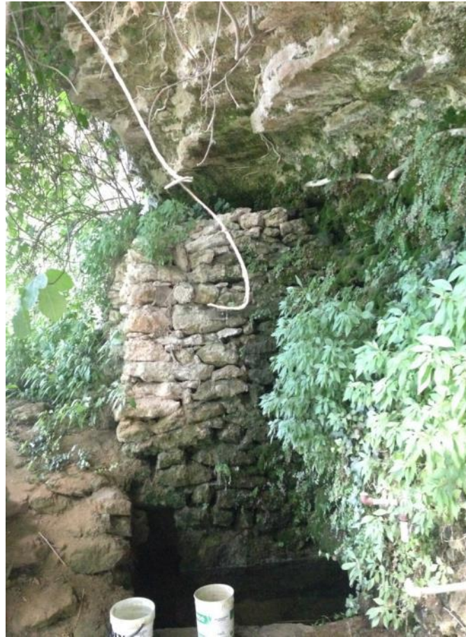
Fig. 17. A dry stone wall interposed between the rocky body and a cistern in the Orti Saraceni.
