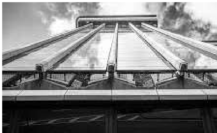
60. Bottom view of finished facade.
