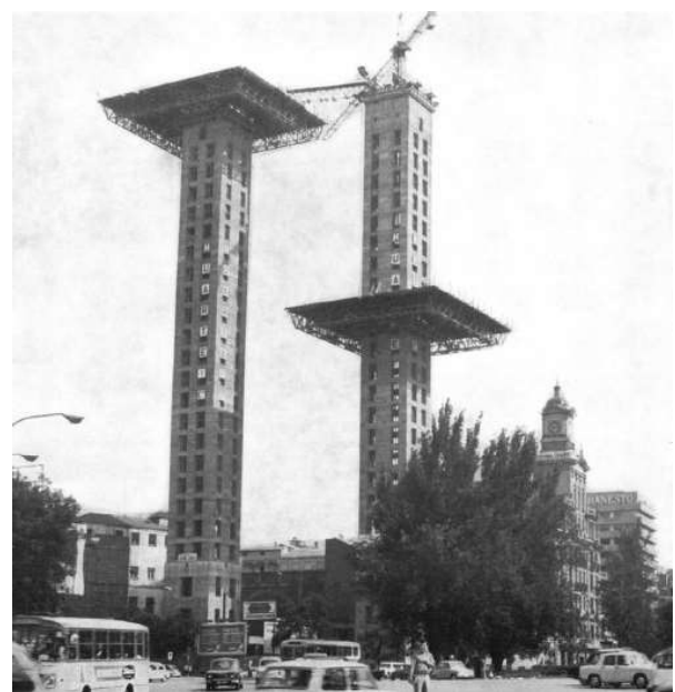
51. Lifting of the framework by bars and climbing jacks.
