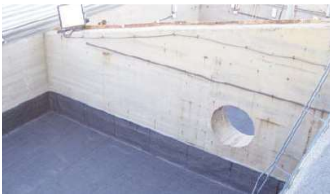
46. Large deck beam
