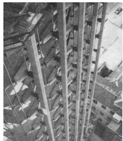
69. Tie rods attached to forged, top view.
