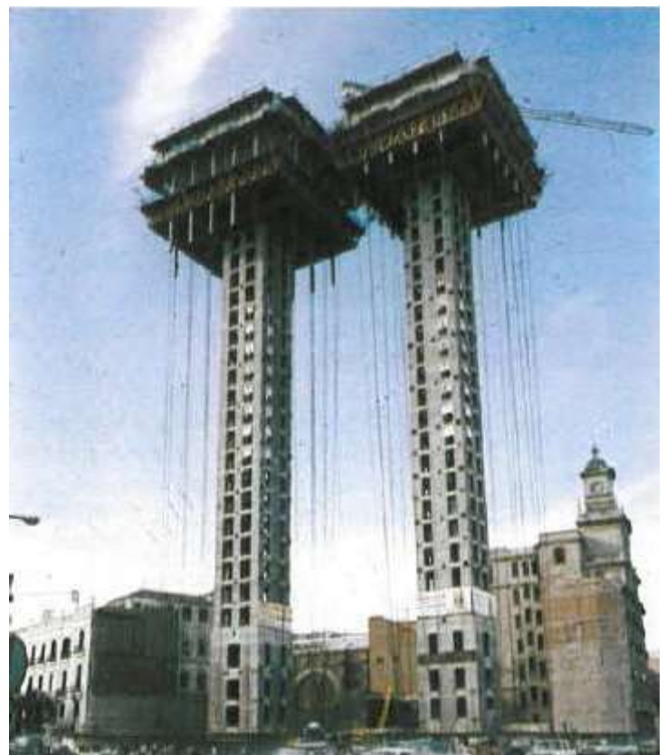
10. Construction of towers plants up to down
