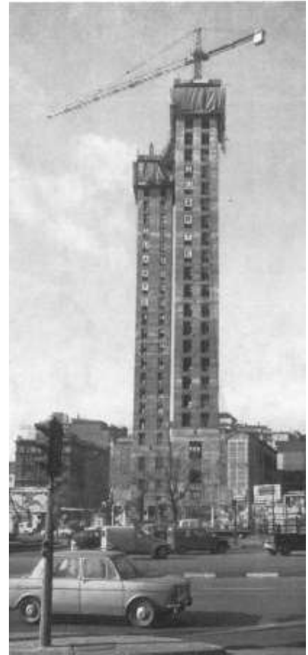
19. Central Core of the “Torres de Colón”
