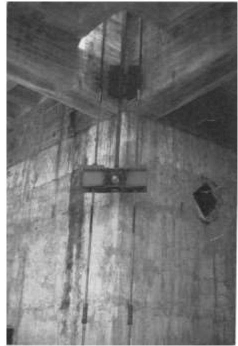
53. Detail of the hanging bar of the formwork.
