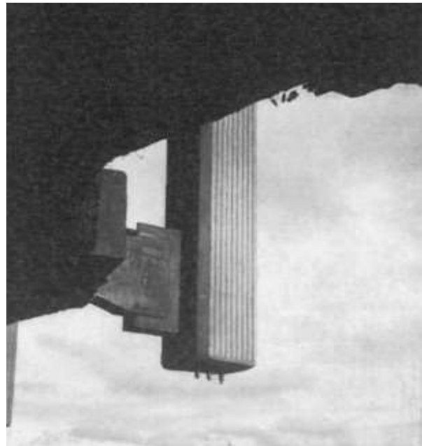
67. Tie rods attached to forged bottom view.
