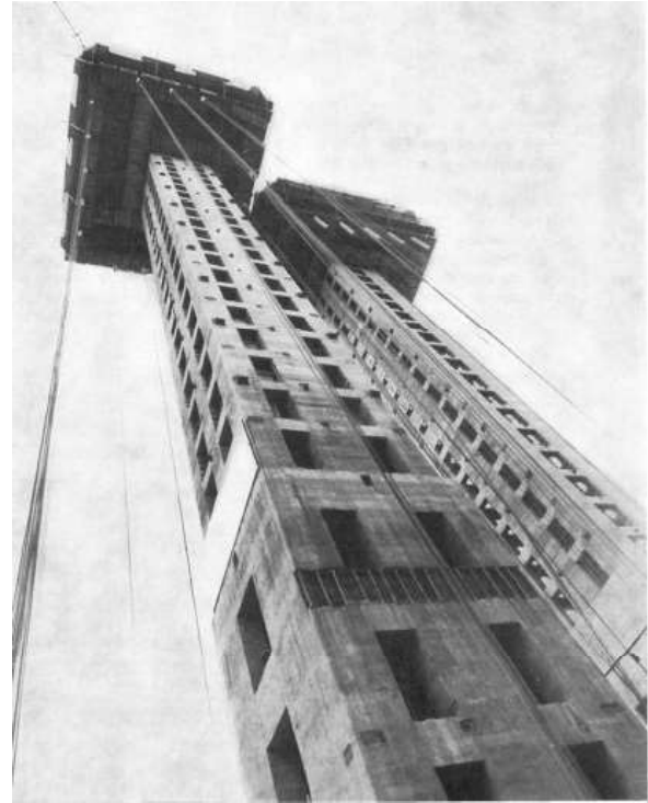
57. Bottom view with suspended tie rods.
