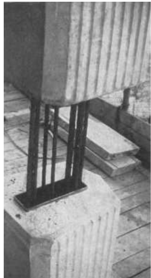
61. Joining of prefabricated tie rods
