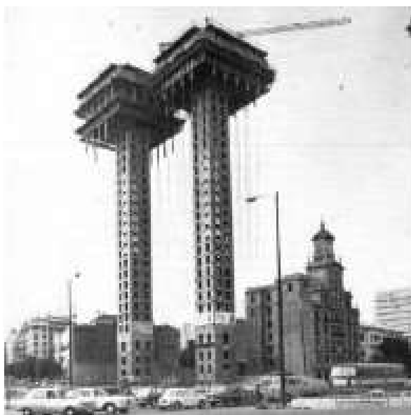
21. Execution of the different plants by tie rods
