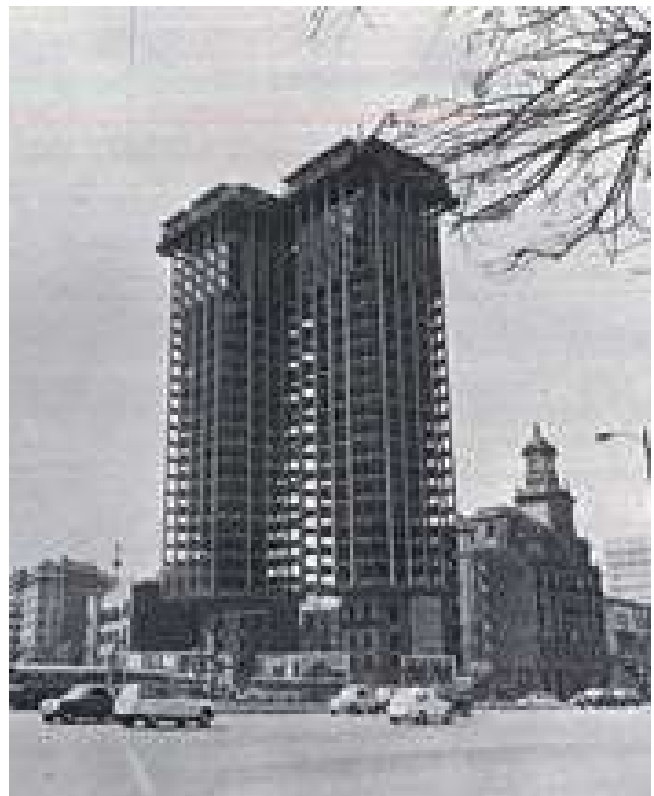
14. Construction of the “Torres de Colón”
