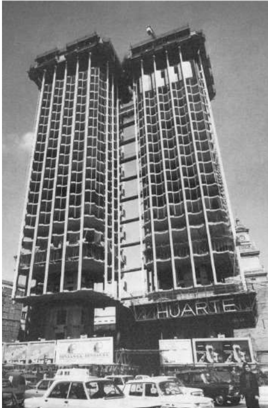
65. Construction of the lower floor.
