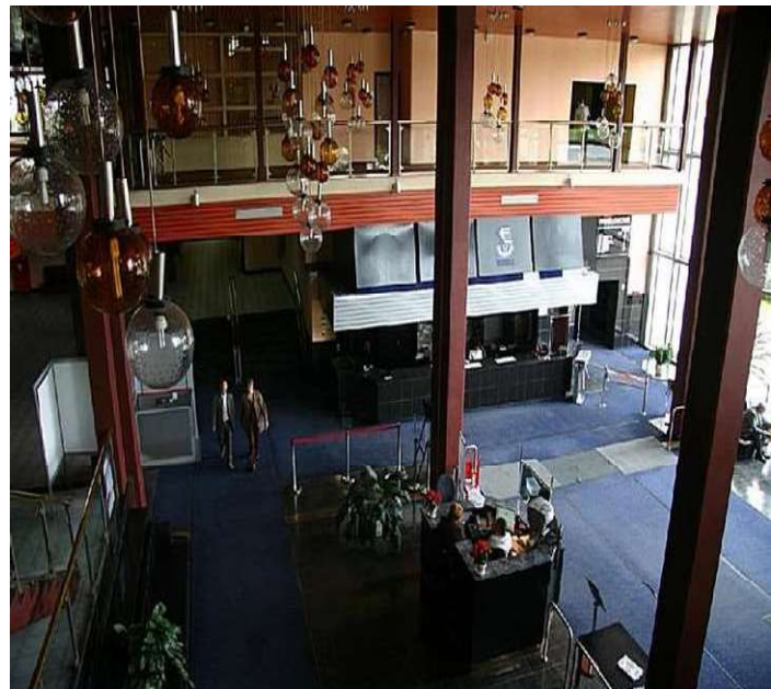
4. View of the low floors of towers Stalexport.
