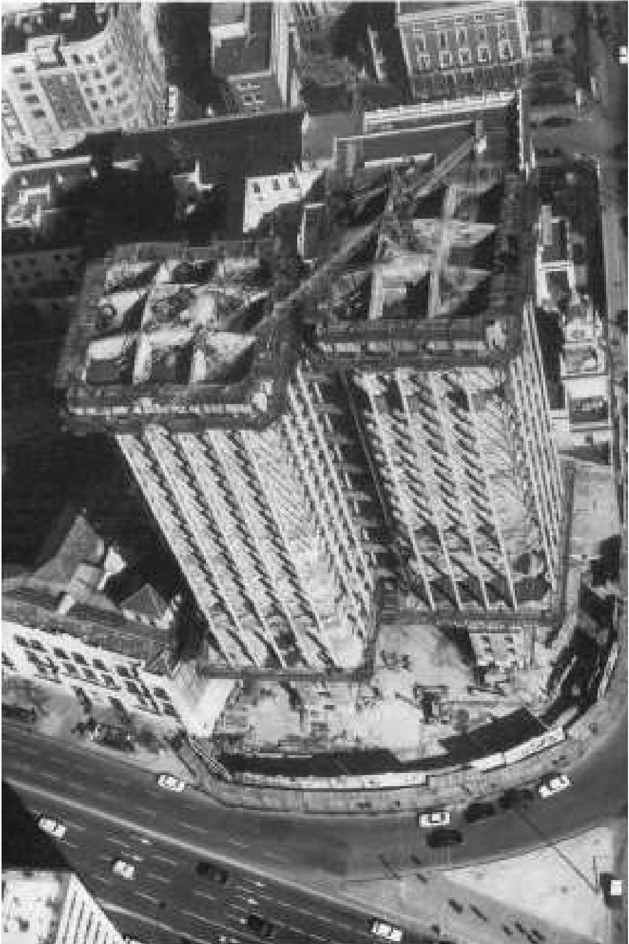
49.b) Execution of the head beams
