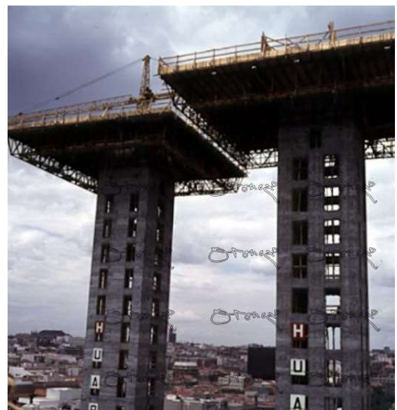
56. Support-formwork platform.
