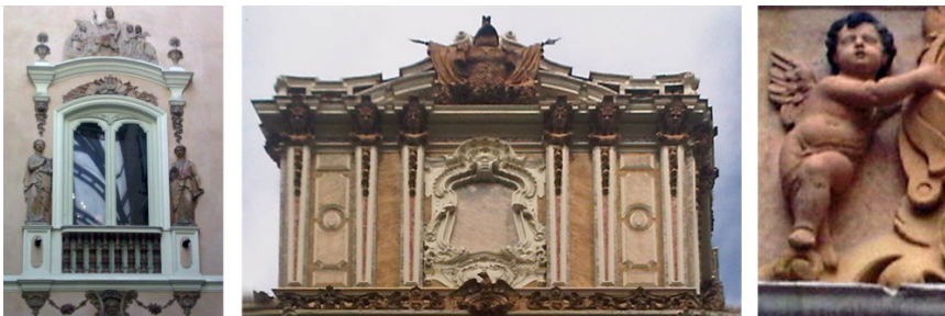
Figure 6: Terracotta details: Marques de dos Aguas Palace and Communion Chapel in St. Martin Church (Cristini; Ruiz-Checa).
