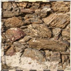
Fig. 4- Masonry sample of Trabuccato tower (Murru, 2014).
