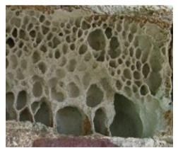
Fig. 6- Alveolation with different size of alveoli (15-80 mm) with lightly iso-orientation, related to different welding inside the same ashlars.
