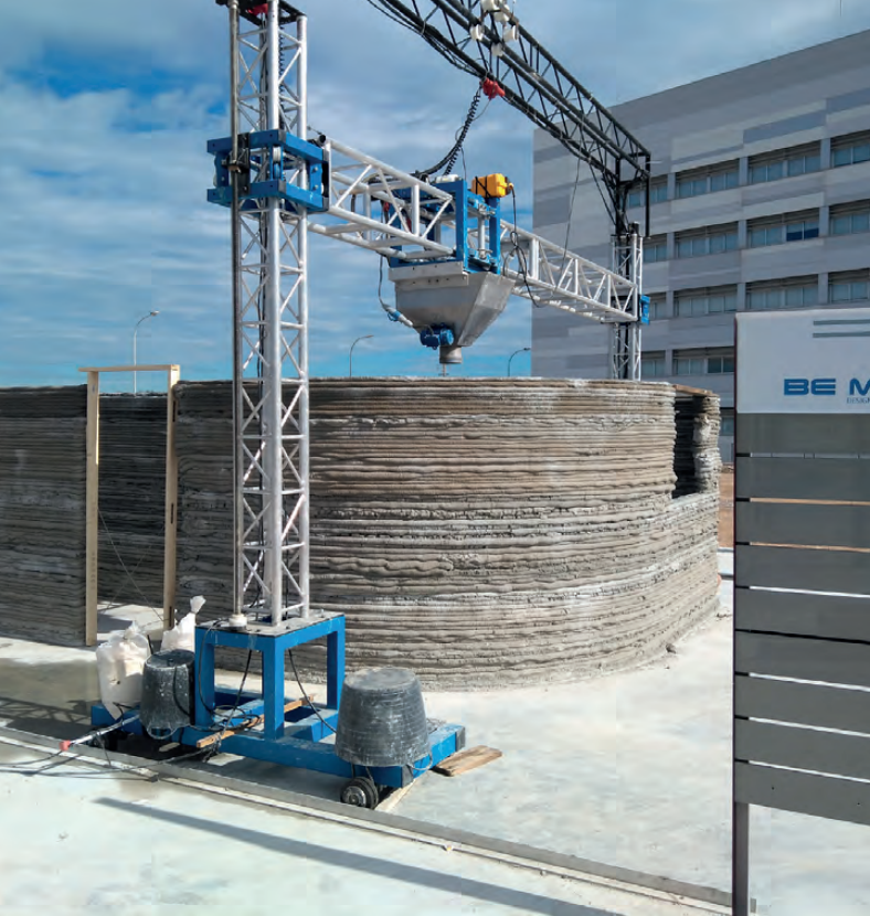
Figure 8. Modelo real casa impresa 3D. BEMORE3D (2018). / Figure 8. Real model of printed house 3D. BEMORE3D (2018).
