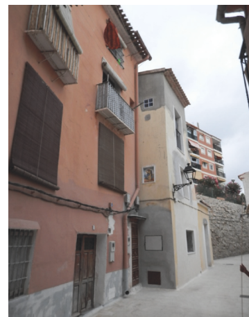
FIGURE 6: Real facade where measurements were taken.
