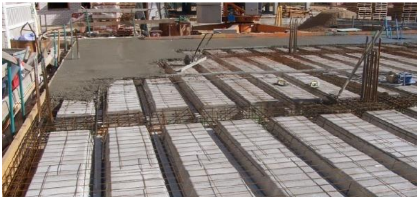
Fig. 6 Wide beams and one-way reinforced concrete floor
